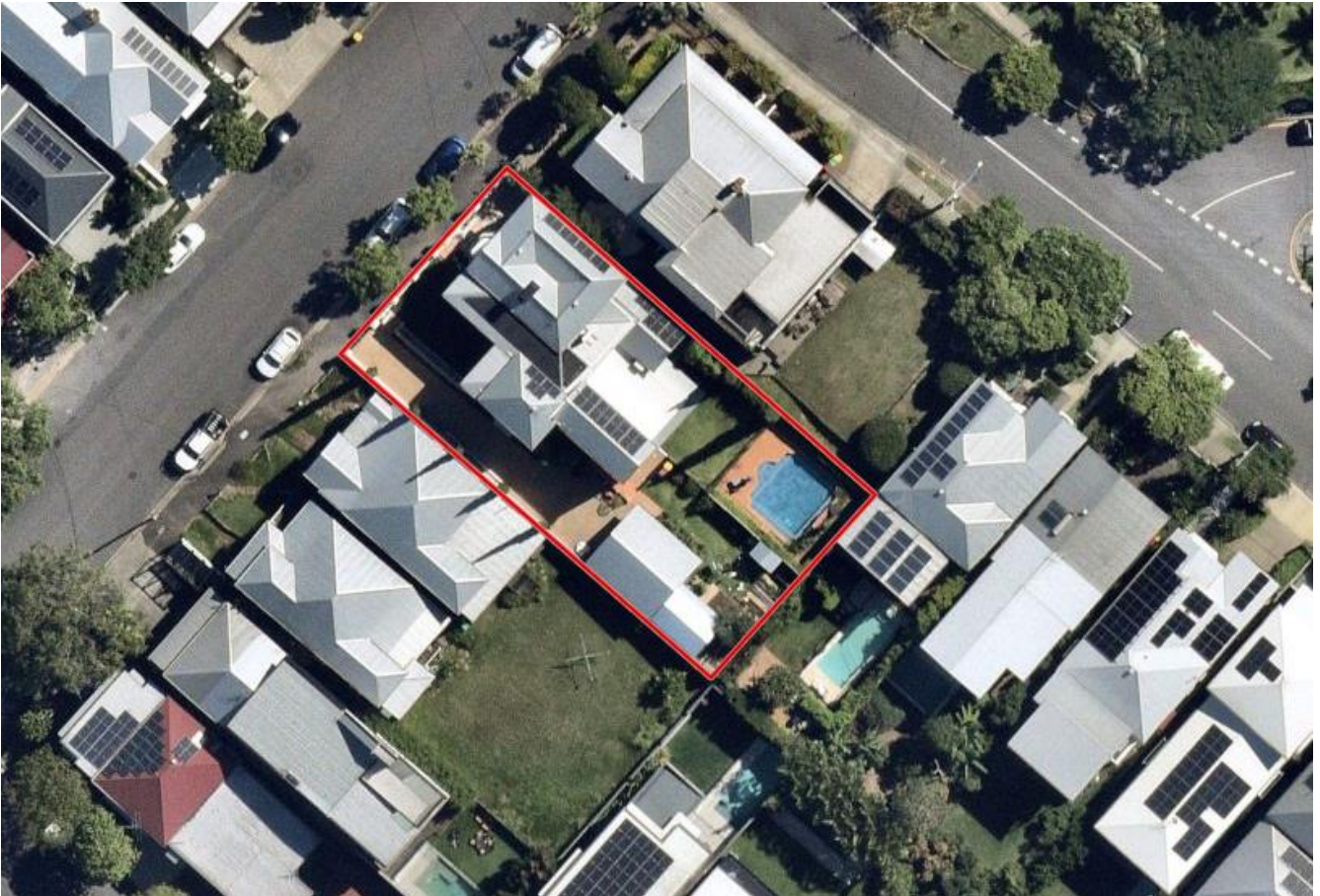
Figure 1- Aerial photo of subject site (Source: Nearmap)
