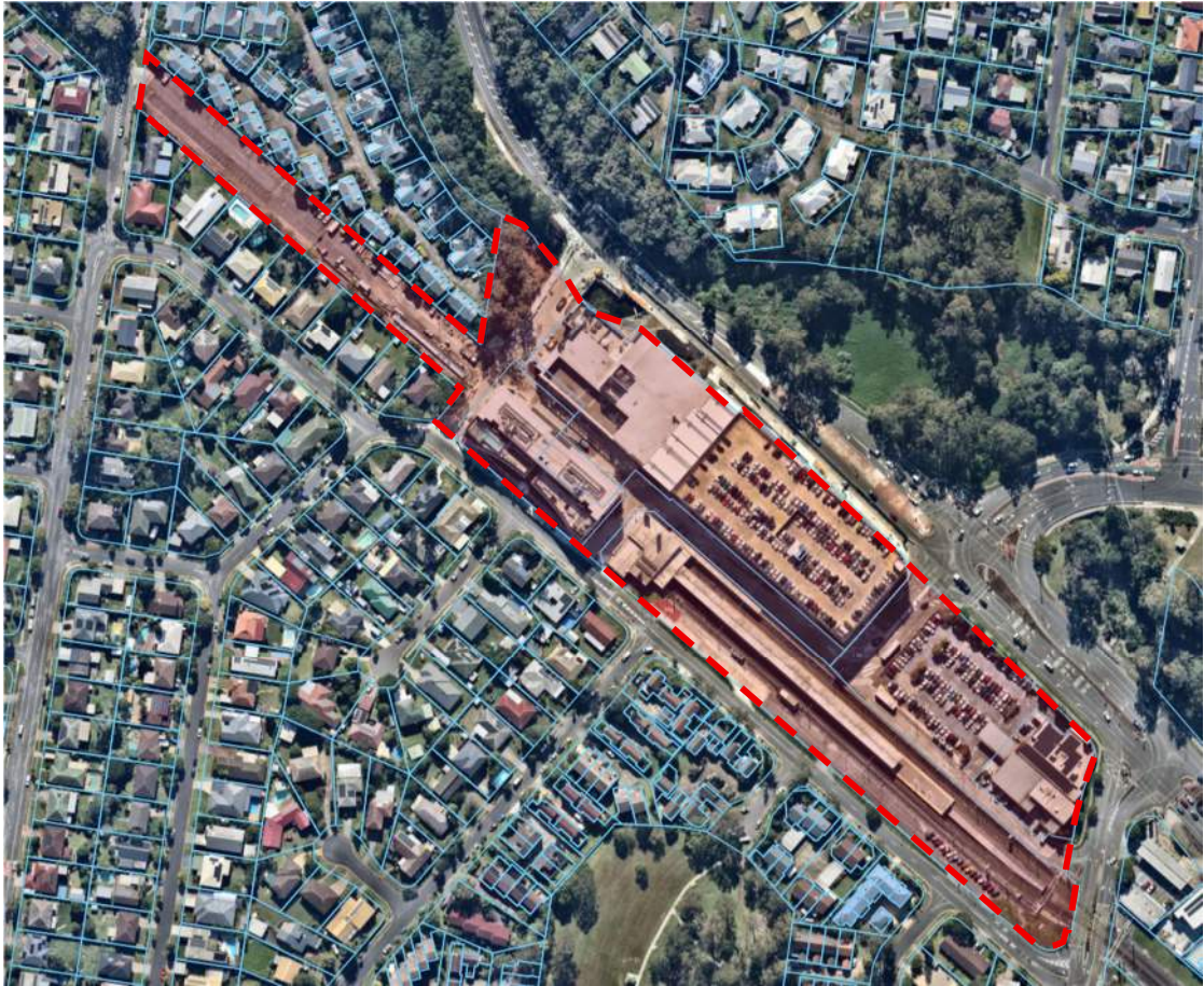
Figure 2 Site Aerial Photograph Source: Near Map, June 2026
