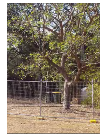
03 FIGURE 3 TPF1 xx01 1800mm high steel mesh fence. Installed following survey setout fence to be supported and clamped.
