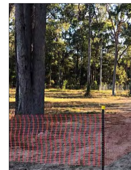
04 FIGURE 4 TPF2 xx01 Orange mesh with steel staking to be used in support locations and where ground conditions limit the access for TPF1. Fence line to be based on surveyed positioning.
