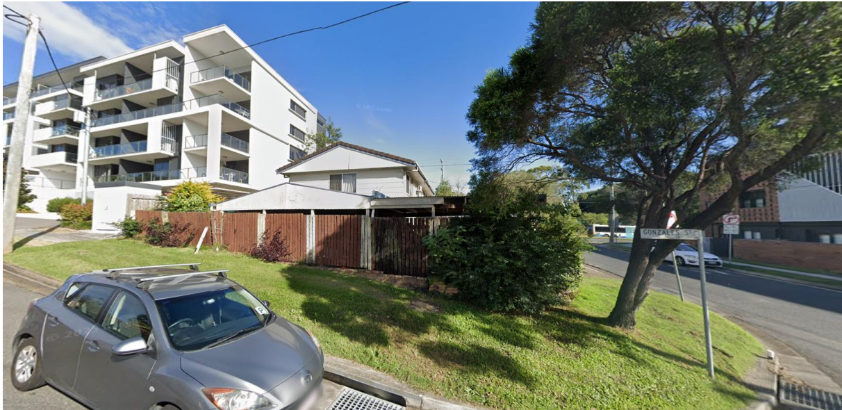
Figure 2-4 Gonzales Street Frontage
