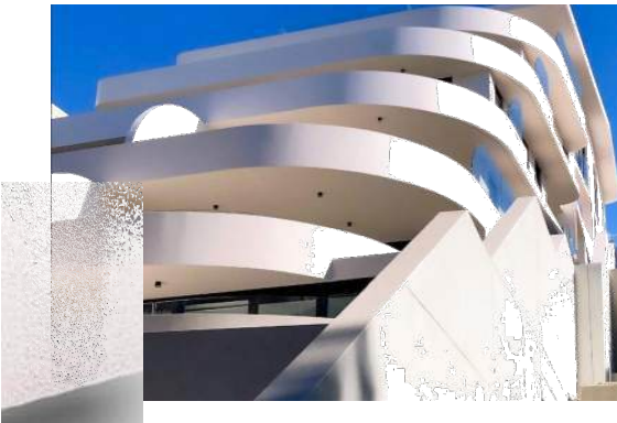
RENDERED BLOCKWORK PAINT FINISH
