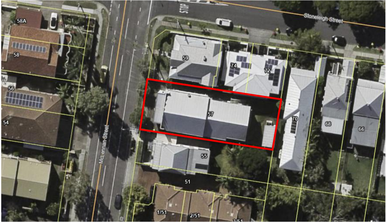
Figure 1: Aerial image of the application site (in red) and surrounding area. Source: Queensland Globe.
