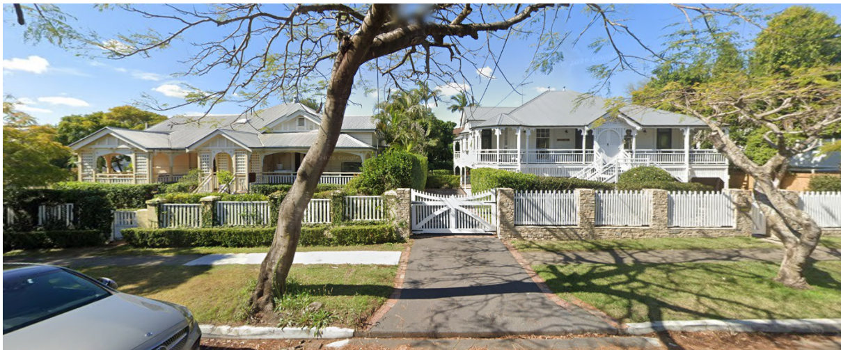
Figure 8: 49 and 51 Charlton Street, Ascot adjoining 112 Racecourse Drive along the rear boundary (west) (Source: Google Maps, 2026)
