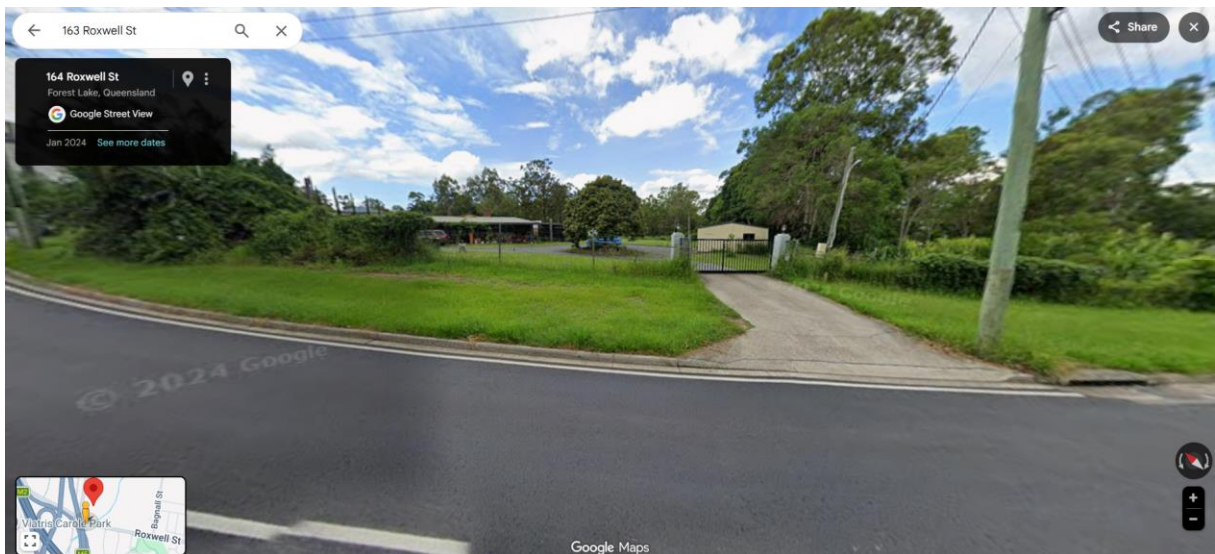
Figure 2-2 Site Viewed from Roxwell Street
