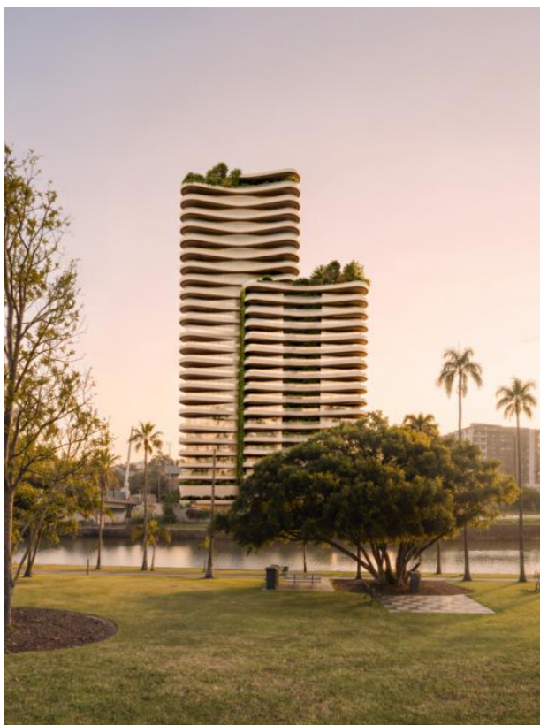
Figure 8: Proposed Sculptural Architectural Landmark with Stepped Building Heights – View from Newstead Park (Source: Kennon – Design Report)
