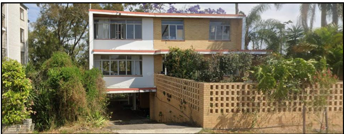
148A Sherwood Road – Google Street View Photo showing an existing post-1946 multiple dwelling with brick walls and flat roof form
