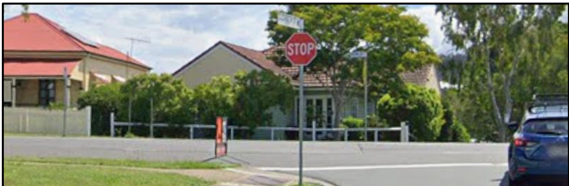
38 Dean Street – Google Street View Photo showing an existing post-1946 dwelling house with rendered walls and tile roofing
