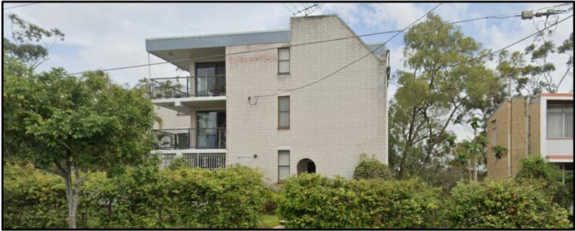
148 Sherwood Road – Google Street View Photo showing an existing post-1946 multiple dwelling with brick walls, flat roof form, and tall glass sliding doors
