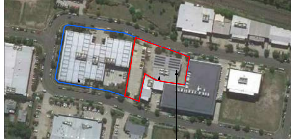
50 + 68 SOUTHGATE AVENUE - AERIAL VIEW
