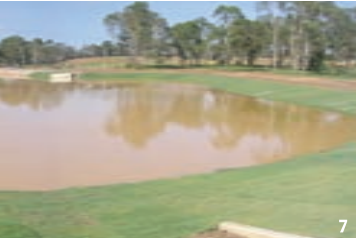
Figure 3 15: Building basin operating as a sediment basin during the building phase
