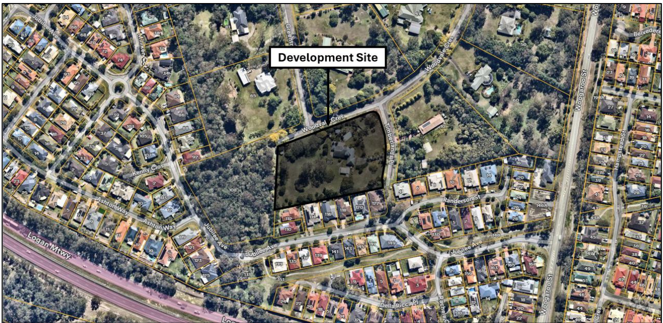
Figure 2-1 Development Site Location (Source: Nearmap, August 2025)
