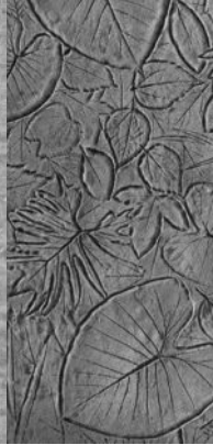
OFF FORM CONCRETE FINISH
