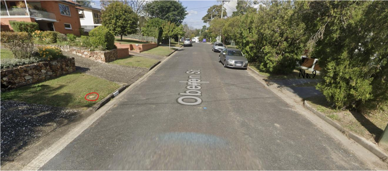
Image : Existing Fire Hydrant Location
