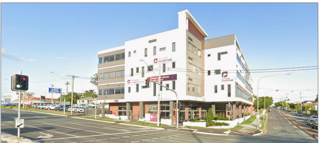
Figure 5: Subject Site viewed from Rode Rd
