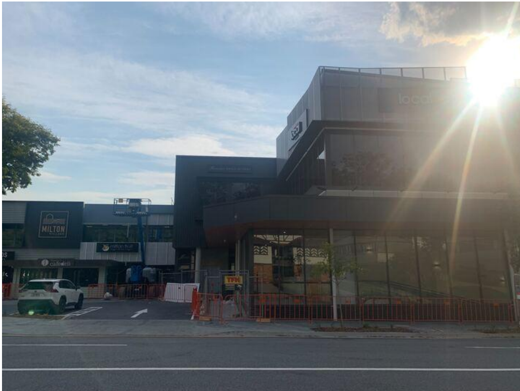
Renovations at Milton Village
