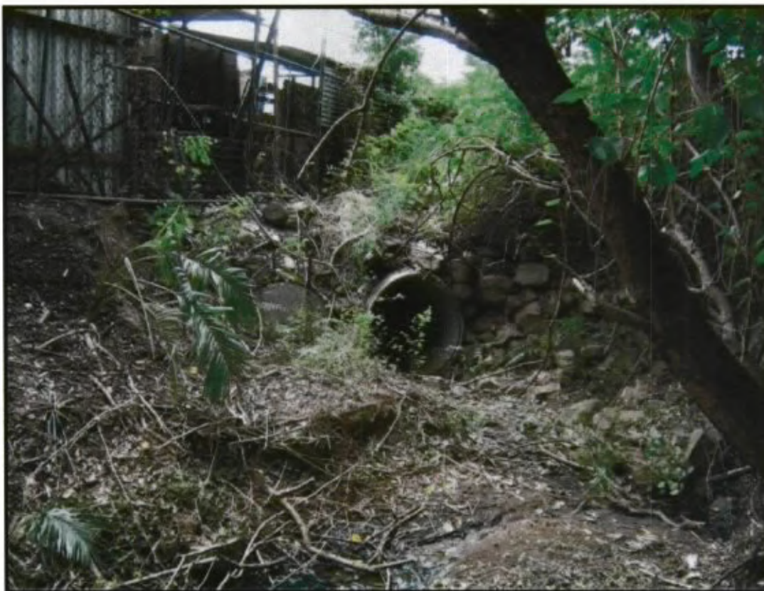
Photo 2 – The inlet works for the 1050mm diameter pipe constructed below 854 Waterworks Rd.
