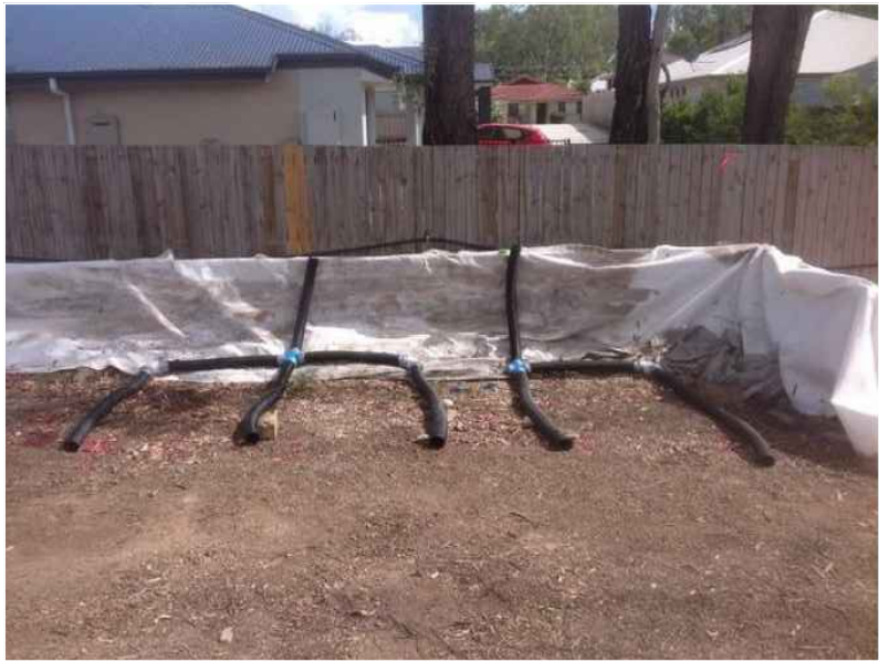
IMAGE 2 (ABOVE). EXAMPLE OF AERATION/MOISTURE TUBE ALIGNMENT
