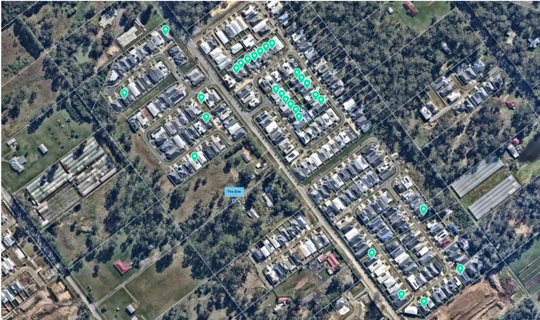
Figure 7-2 Examples of standard lots within the local area and LDR zone that do not comply with the minimum lot width (15m)
