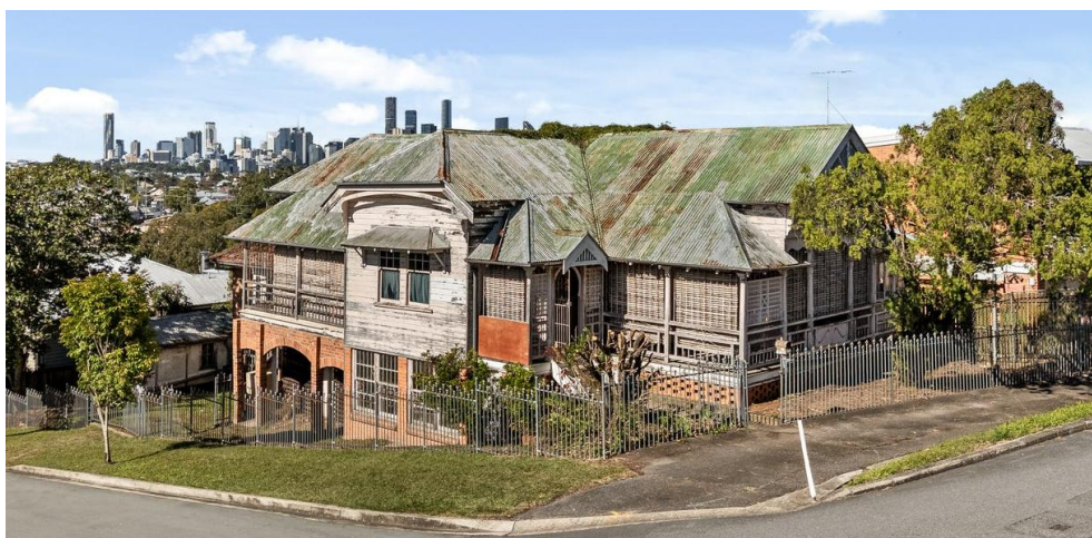
Figure 5: Original timber Dwelling house (View from Corner of tooth Avenue)
