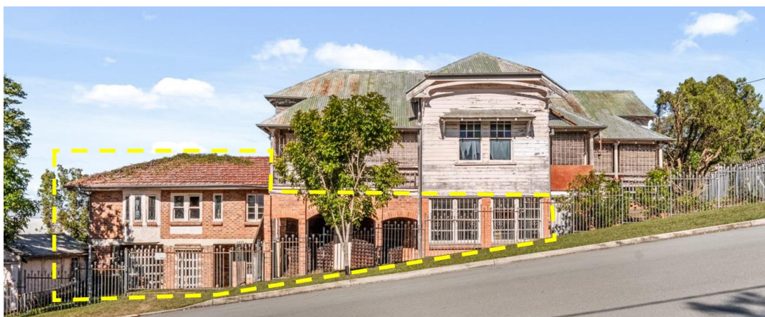
Figure 7: Brick Extension (View from Tooth Avenue)
