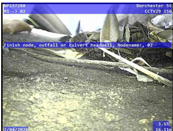
17, 00:08:18, 16.12 Finish node, outfall or culvert headwall, Nodename:, 02
