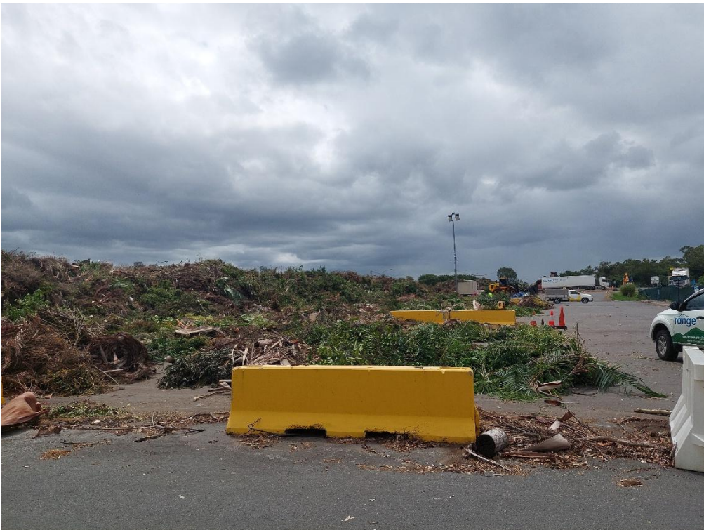
Photograph 4 View to the north of greenwaste pad
