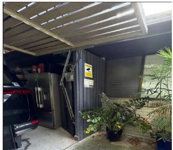
B. Tilt Panel Door at the front of the Garage
