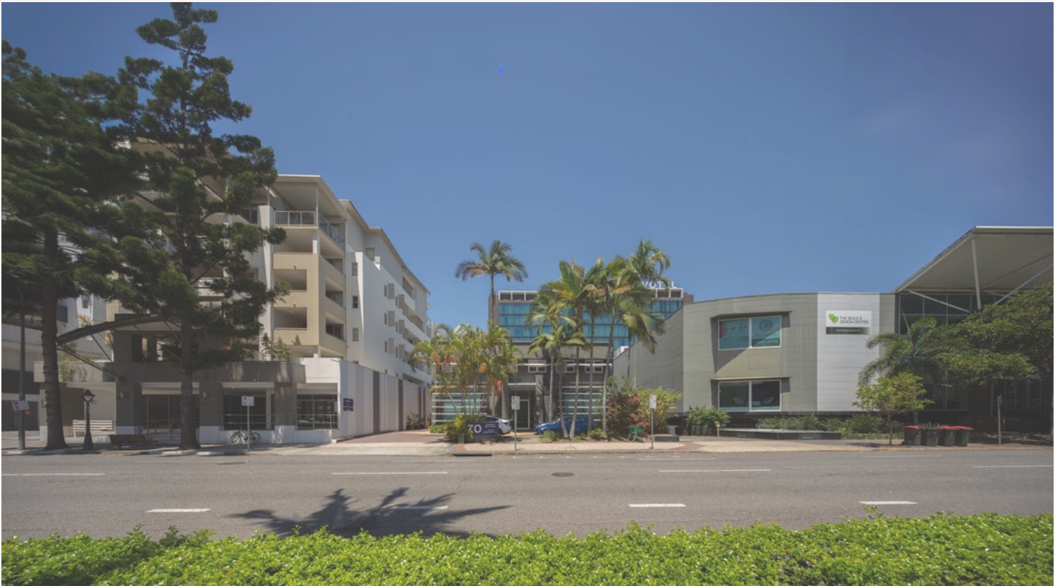
2. Merivale Street Frontage
