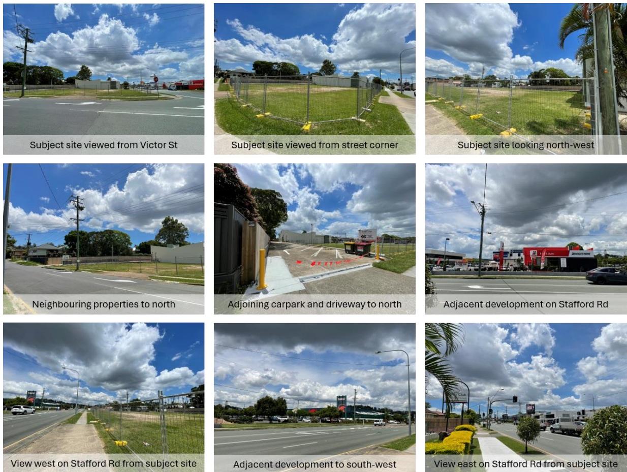
Figure 2: Photos of subject site and surrounds
