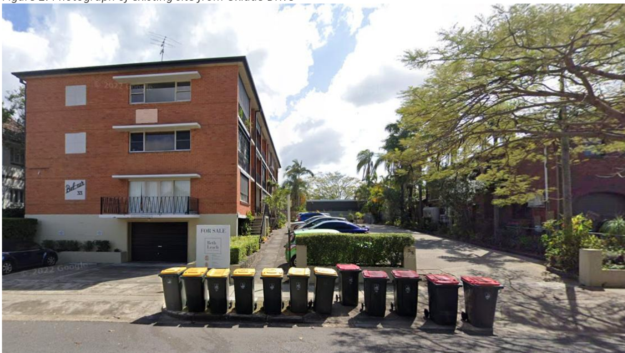
Figure 2: Photograph of existing site from Oxlade Drive
