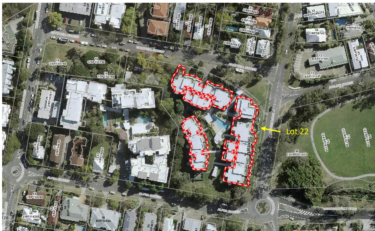
Figure 1: Satellite view of the four buildings in Encore complex and site identification
