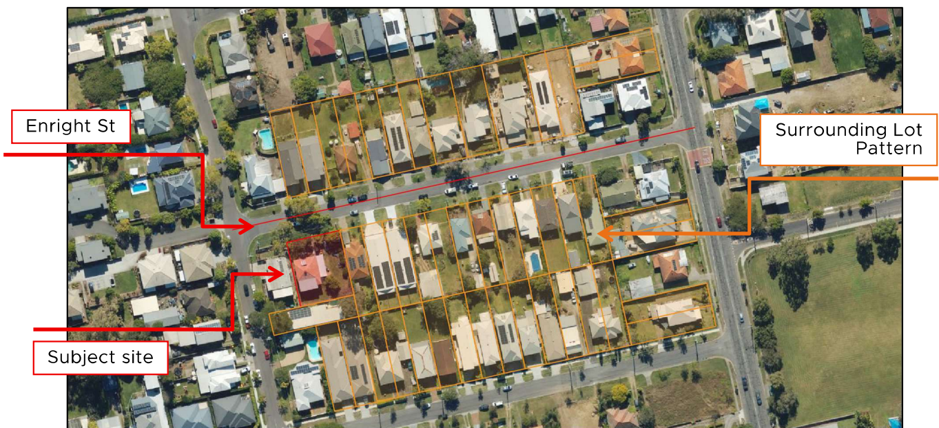
Figure 5: Enright Street Catchment Area - Subject site shown in red. Source: Queensland Globe
