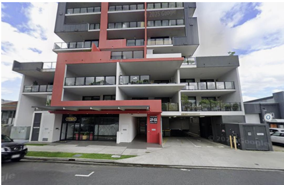
Figure 1: The adjoining development at 33 Nundah Street.
