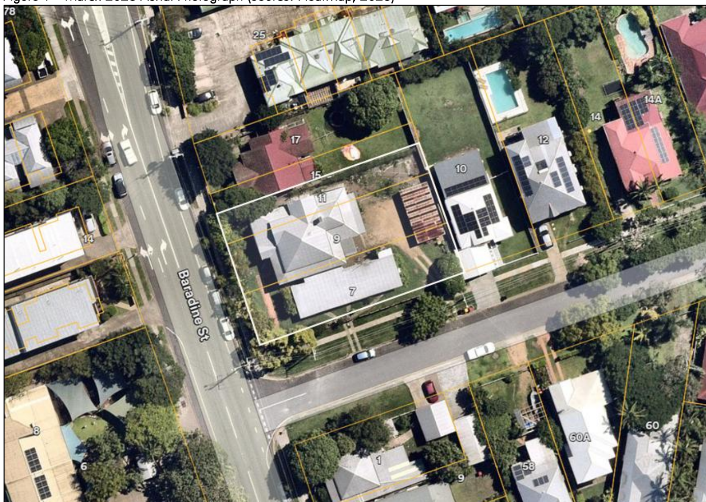
Figure 1 – March 2026 Aerial Photograph (Source: NearMap, 2026)
