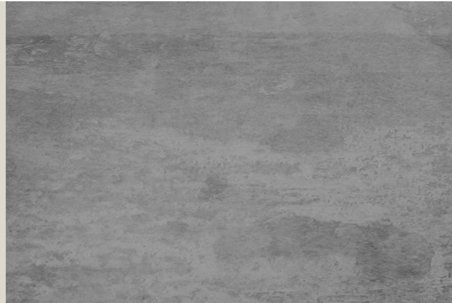
Off Form Concrete
