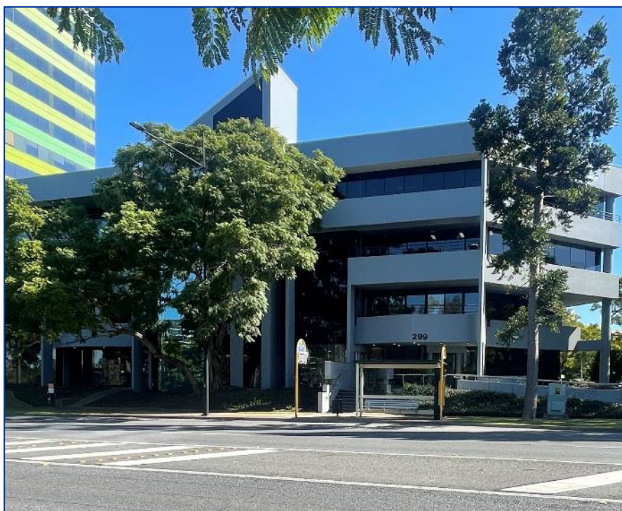
Figure 2.2: View of the Subject Site Towards Coronation Drive
