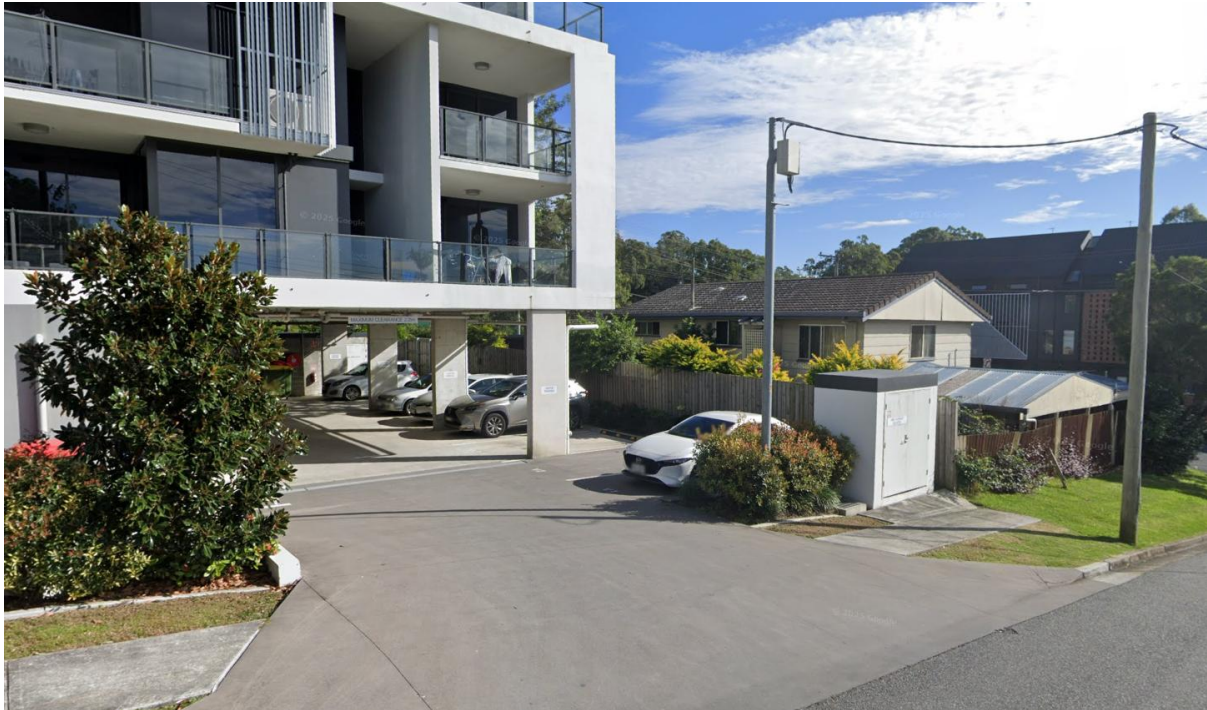
Figure 3 Street View (Gonzales Street) of the Site and adjoining site to the south
