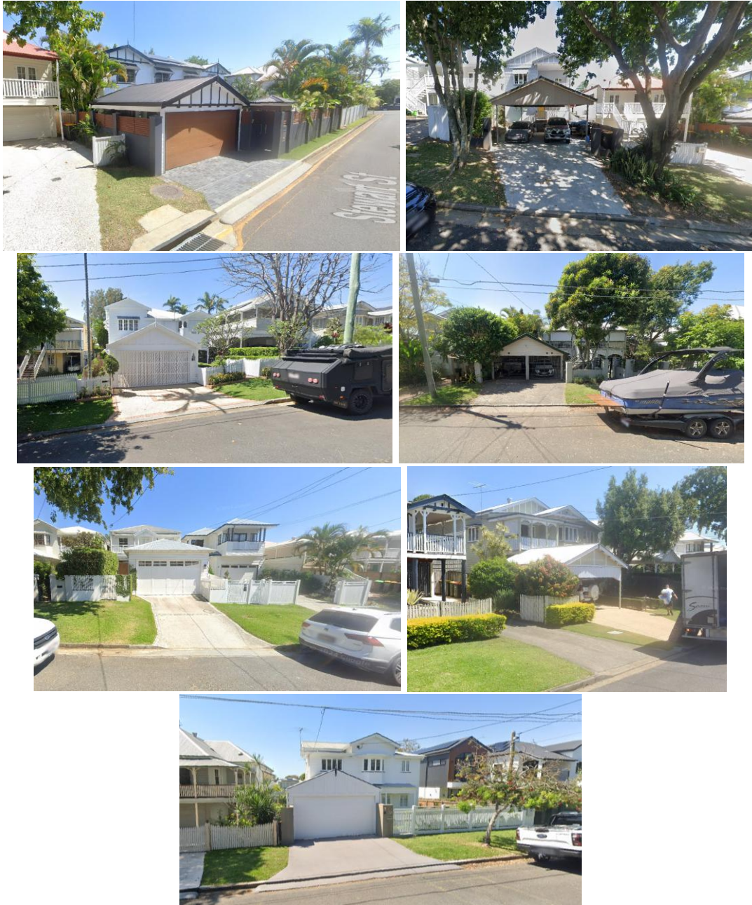
Figure 14: Double carports and garages forward of the building line located on Stewart Street.
