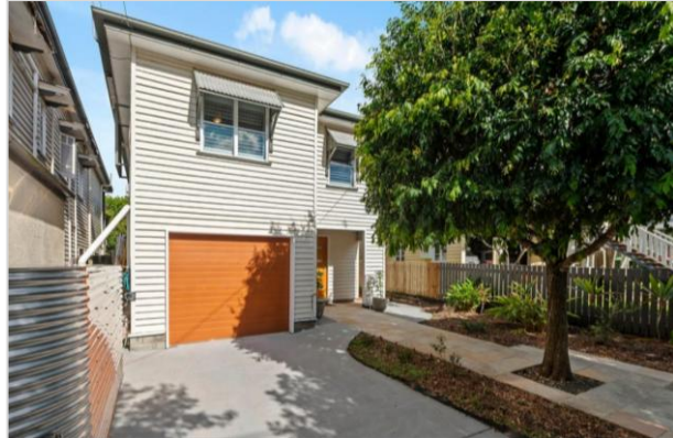
Figure 5: Existing site as viewed from Stewart Street (3).
