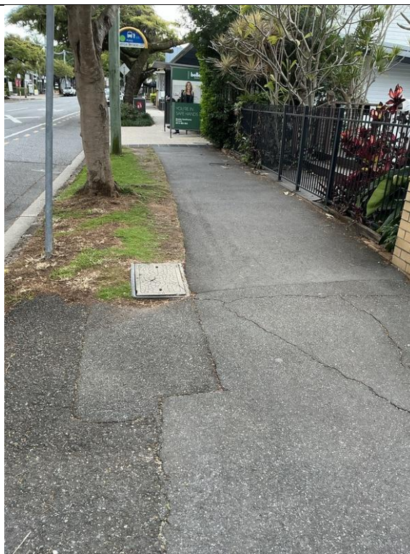
Photo 4. Footpath Demolition. Image C. Anglesey
