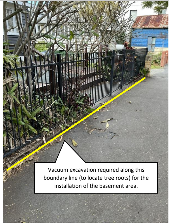
Photo 6. Basement Excavation. Image C. Anglesey
