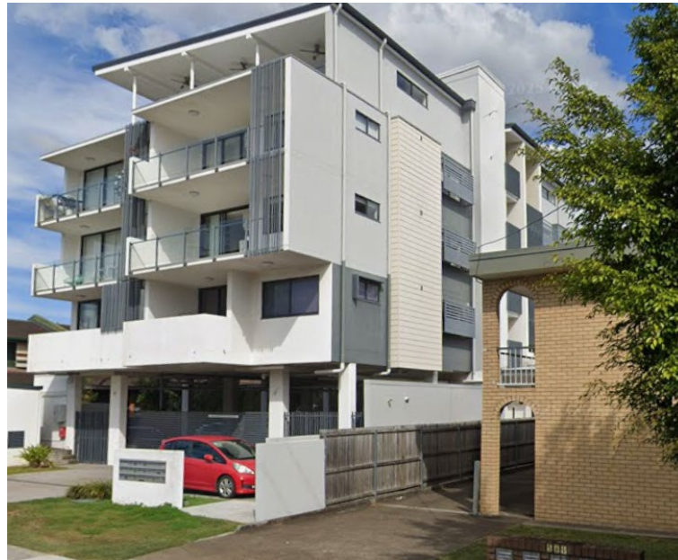
Figure 21: Existing screening outcomes - 564 Sherwood Road, Sherwood (Source: Google Maps, 2026)
