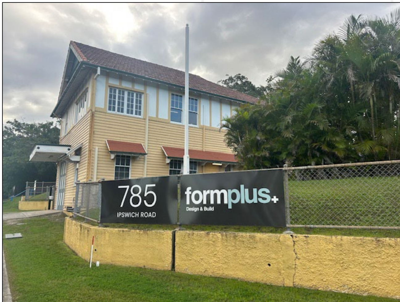
Figure 3: Corner of Ipswich and School Road
