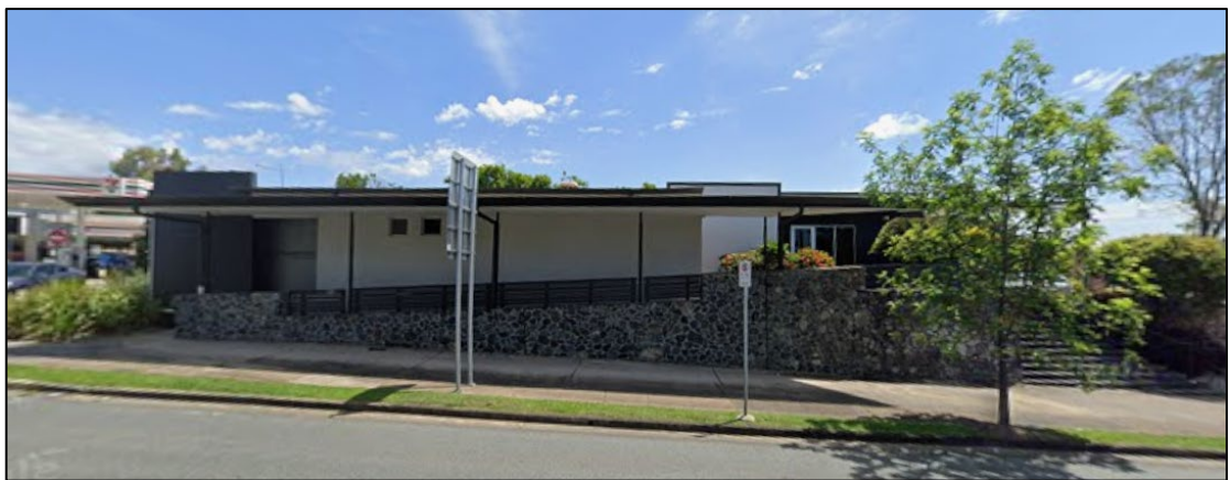
Figure 3 - Subject Site as viewed from Samford Road
