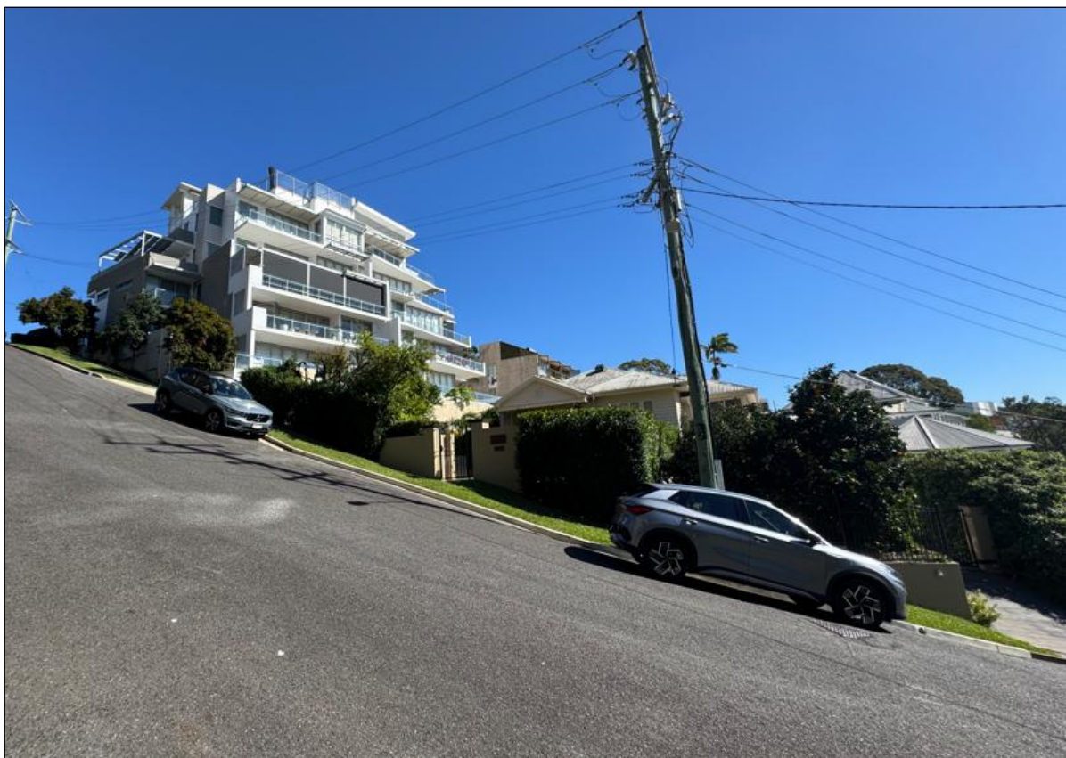
Figure 5: Site Photograph. Image of the Subject Site (21 Kings Road) as viewed from the Kings Road frontage.
