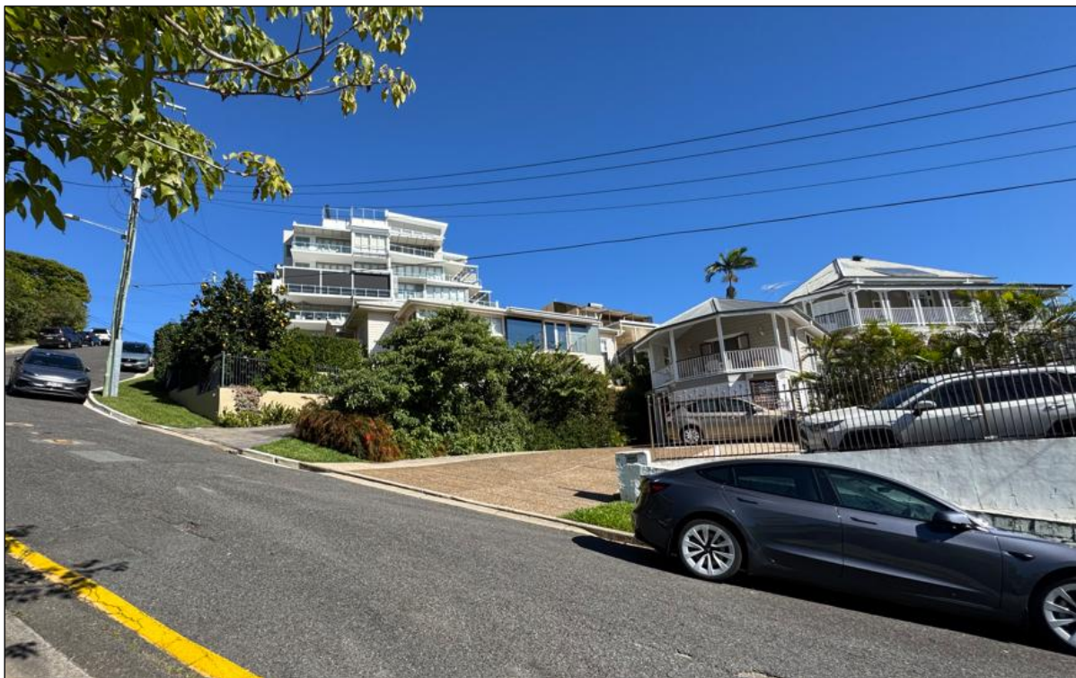
Figure 3: Site Photograph. Image of the Subject Site (11 Kings Road) as viewed from the Kings Road frontage.
