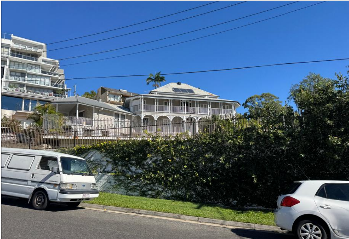
Figure 2: Site Photograph. Image of the Subject Site – (11 Kings Road) as viewed from the Kings Road frontage.
