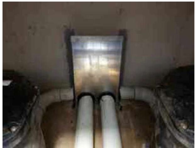
Figure 3 - Typical Outlet Weir Wall
