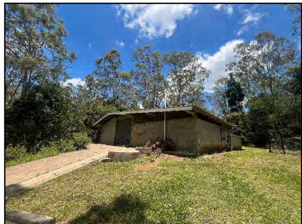
Plate 2 Shed located within proximity to proposed BLE 3.
