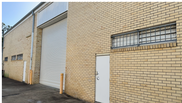
Figure 2: Site photograph of existing western side elevation and the main entry door and roller door opening providing access to customers. Note that no changes are proposed to the existing external facades with the exception of signage in accordance with Council's Local Law.
