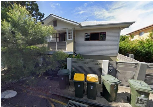
Picture 1: Adjoining 2-storey multiple dwelling at 153 Terrace Street (eastern site boundary)
