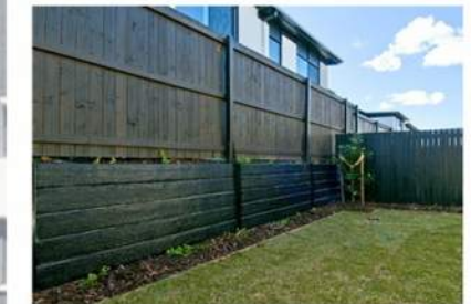
02 INDICATIVE IMAGERY 1800mm HIGH TIMBER PALING FENCE TO REAR / SIDE BOUNDARY - WITH STEP DOWN WHERE REQUIRED.
