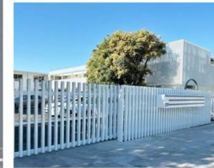
01 INDICATIVE IMAGERY OF 1800mm HIGH ALUMINIUM BATTEN FENCE PAINTED WHITE (50% TRANSPARENCY) TO FRONTAGES
