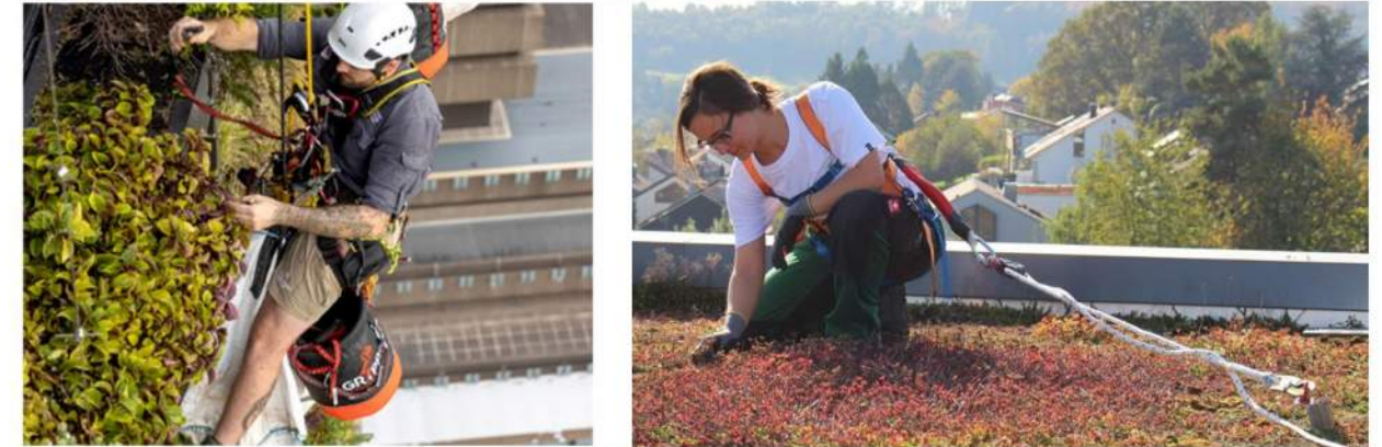
MAINTENANCE ACCESS DETAILS FOR PODIUM PLANTERS TO BE FINALISED DURING DETAILED DESIGN PHASE . INDICATIVE IMAGES OF TWO MOST COMMON APPROACHES: ROPE ACCESS VIA ROOF AND FALL ARREST SAFETY ANCHORS WITHIN PLANTER BOXES
