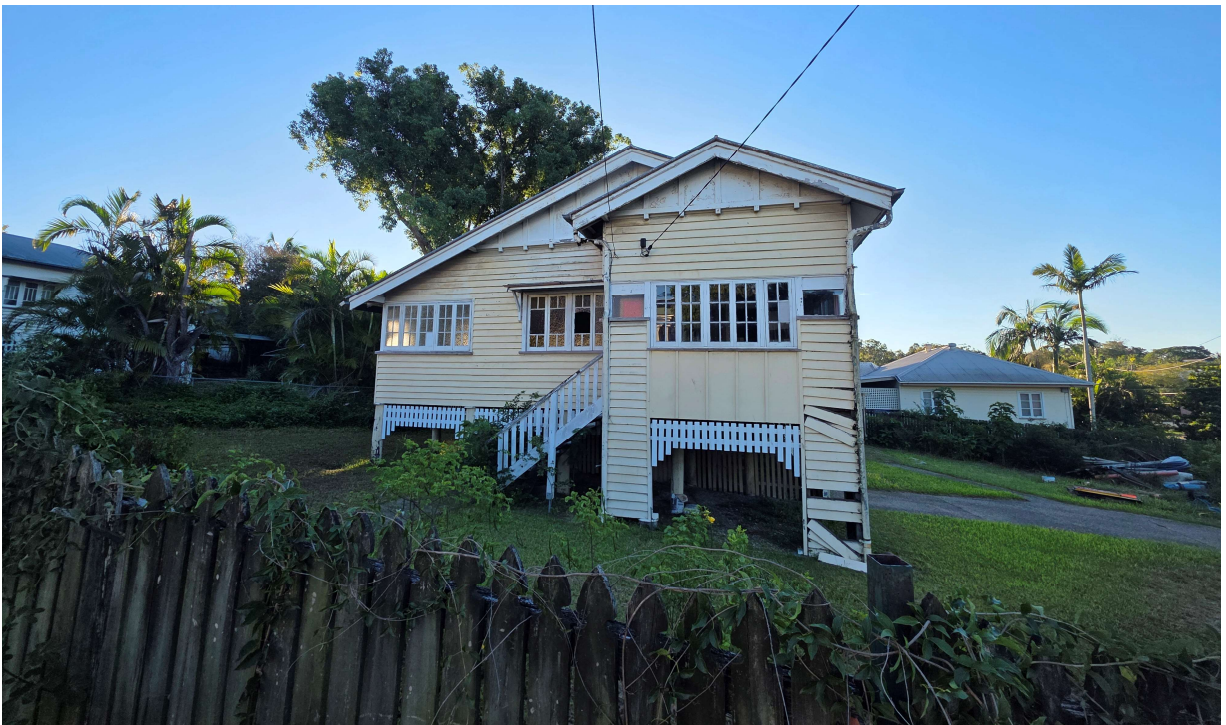
Image 10 – Adjoining pre-war house on 30 Holland Road (Source: Site Visit)
