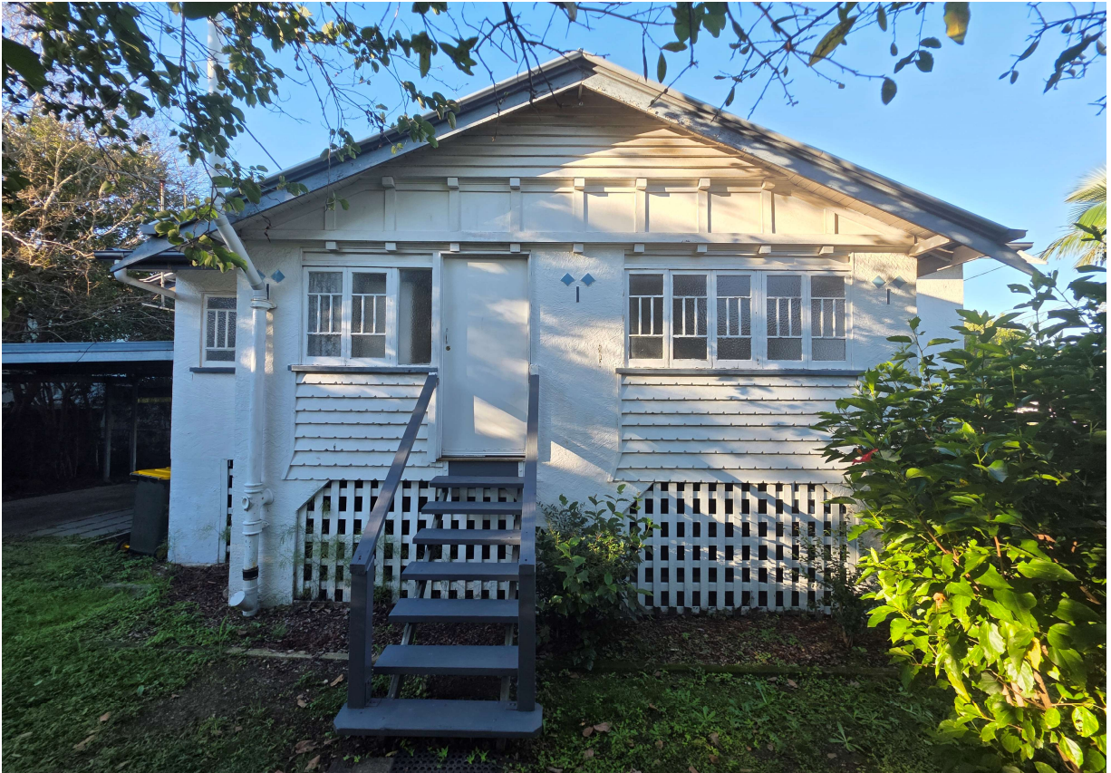
Image 05 – Existing house – West Elevation to Contay Street frontage (Source: Site Visit)
