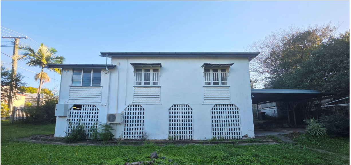
Image 07 – Existing house – East Elevation (Source: Site Visit)
