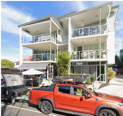
Figure 12: 15 Fox Street Front Façade
