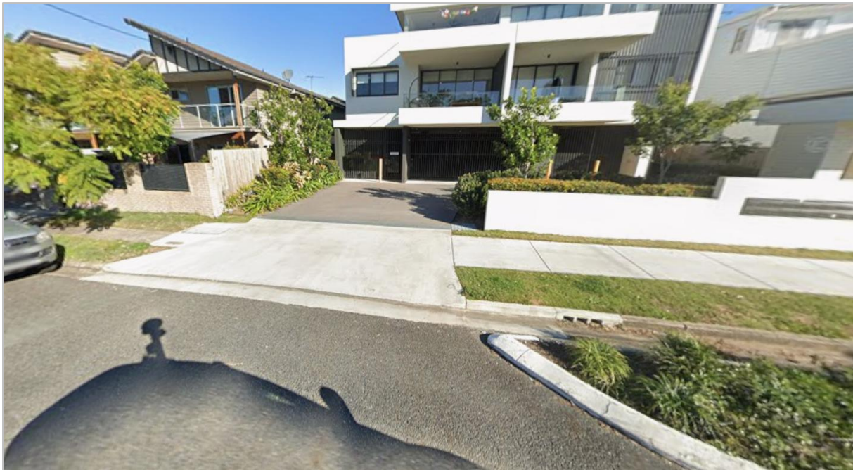
Figure 3.1: Driveway to Development Opposite at 37 Kates Street
