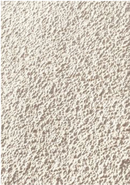
RN-01 Warm-coloured shotcrete look textured render
