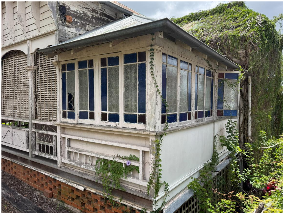
Figure 7: Existing south-western corner
